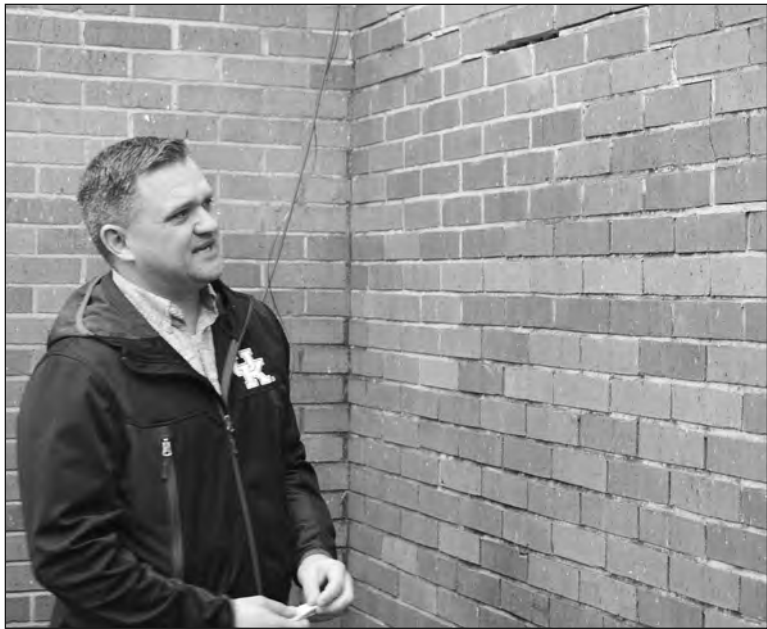
Settling of the foundation since the National Guard Armory in Marion was constructed in 1963 has created numerous problems at the facility on Rochester Street. Above, Kenny Staley, facilities manager for Kentucky Army National Guard, points out a separation of mortar from the bricks on the exterior of the building. At top right, a crack in the drill hall that runs from eye level on one wall to the ceiling on another is one of the more noticeable problems to the average onlooker, while more of the same can be seen in a restroom.
