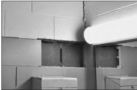
Settling of the foundation since the National Guard Armory in Marion was constructed in 1963 has created numerous problems at the facility on Rochester Street. Above, Kenny Staley, facilities manager for Kentucky Army National Guard, points out a separation of mortar from the bricks on the exterior of the building. At top right, a crack in the drill hall that runs from eye level on one wall to the ceiling on another is one of the more noticeable problems to the average onlooker, while more of the same can be seen in a restroom.
